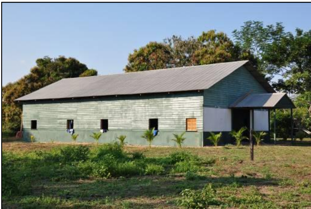
Completed Health Center (Photo Credit: Brian McFarland)
