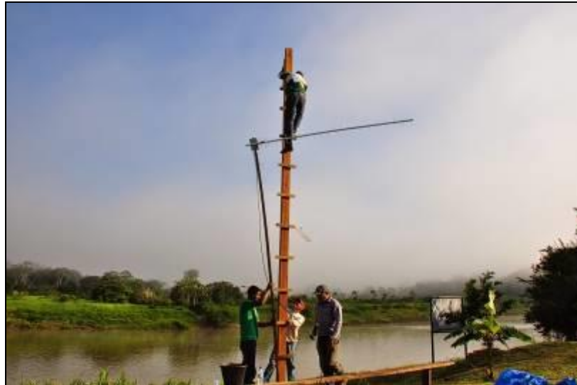
Installation of Phone Tower (Photo Credit: Brian McFarland)
