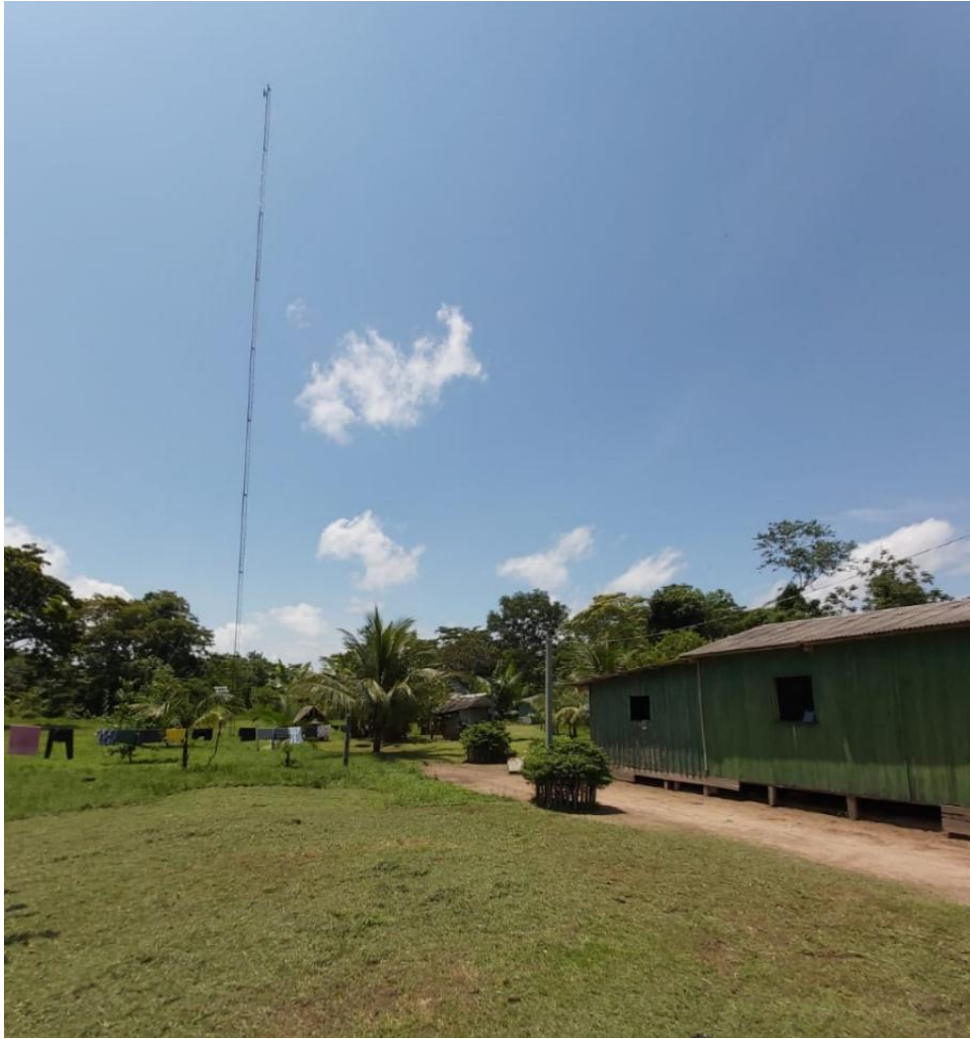
Internet Tower at Purus Project (Photo Credit: Moura & Rosa)
