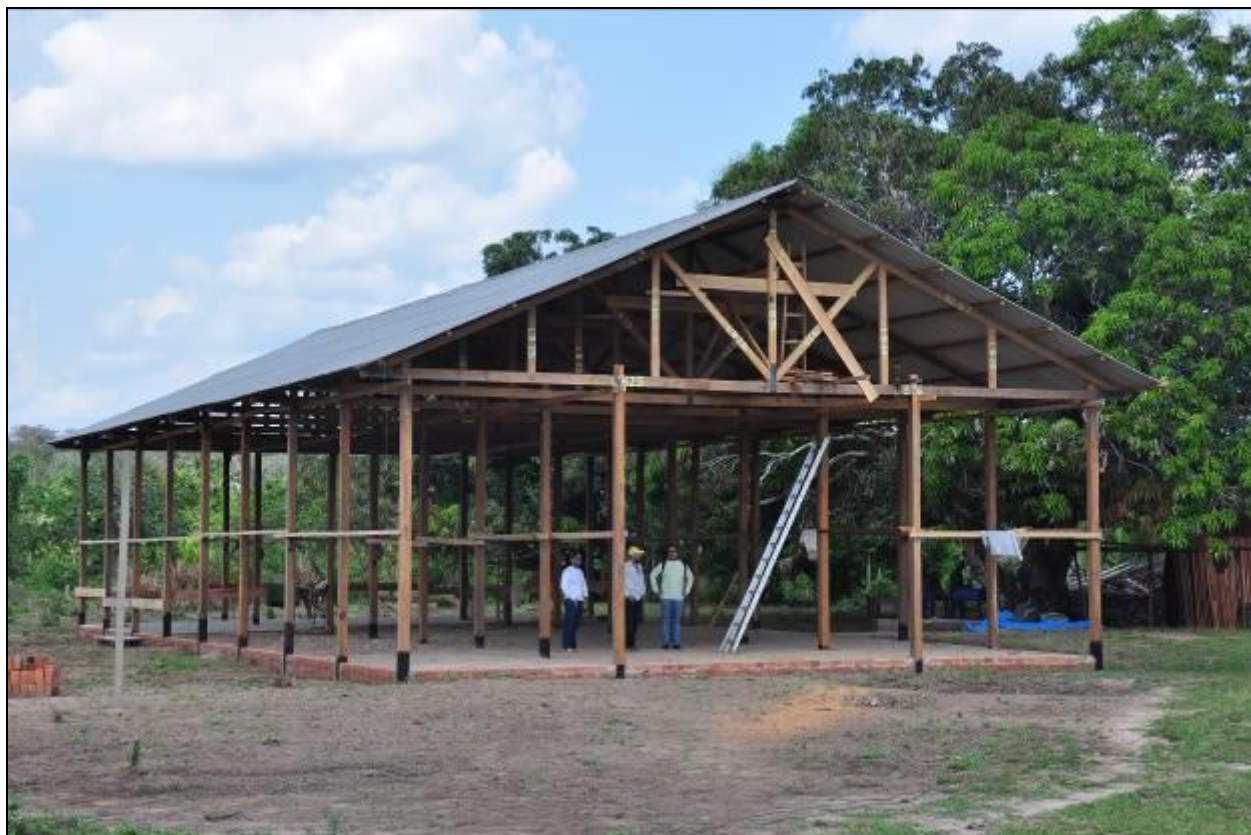
Construction of Health Clinic (Photo Credit: Brian McFarland)
